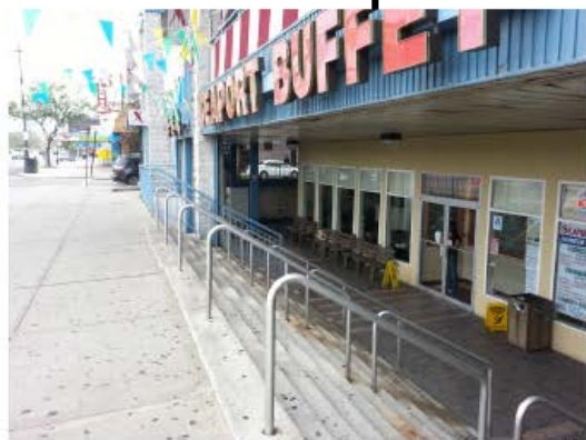
Below grade retail space in cellar
